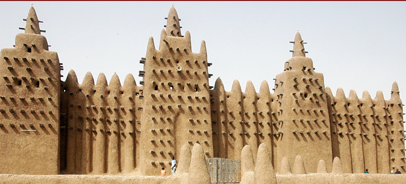
Djenné Mosque in Mali
