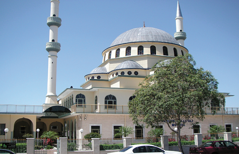
Auburn Gallipoli Mosque, Sydney, Australia
